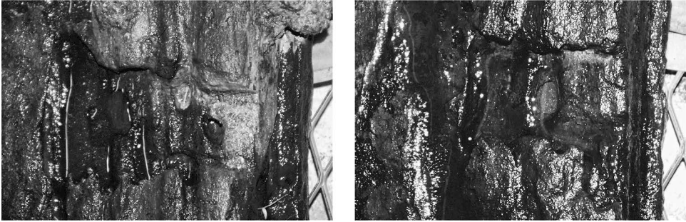
FIGURE 53. Possible dovetail cuts on the bulkhead plank from Takashima. Courtesy of Matsuura Board of Education, photos by author.
